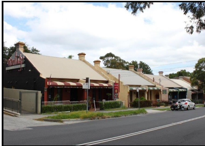
Figure 8: Adjoining development to the west on the opposite side of Dora Street – 35 & 37 Dora Street
