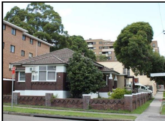
Figure 5: Existing Salvation Army building facing Dalcassia Street – to be retained
